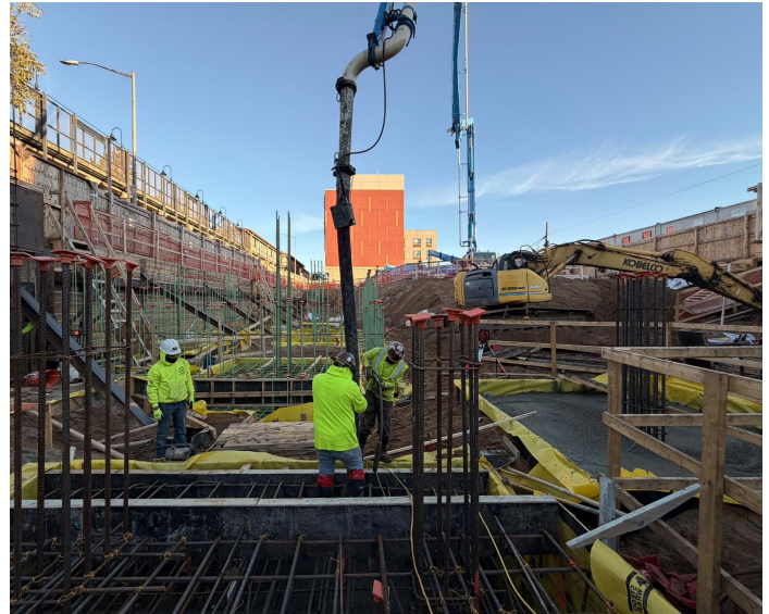
Construction workers at 729 Van Sinderen
